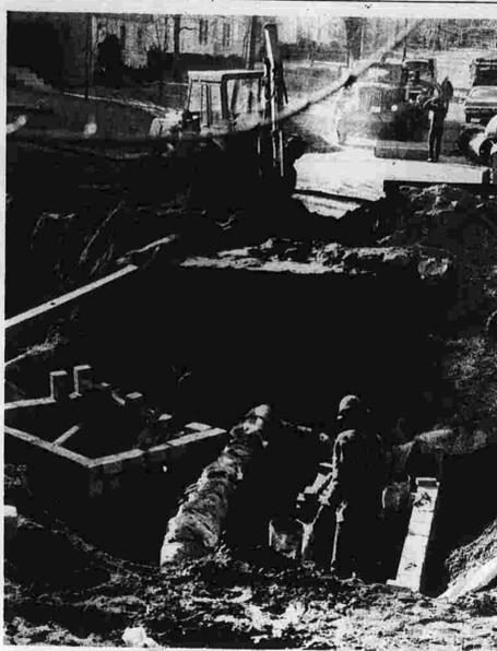
J.N. Clapp Co. crews work on storm drain in the N. Elm St.-White Brook area. The brick structure at left is a storm drainage manhole for the new 48-inch drain. To the left of the workman is a new 10-inch water line owned by the privately owned Manchester Water Co., which serves the area. (Herald photo by Pinto)
