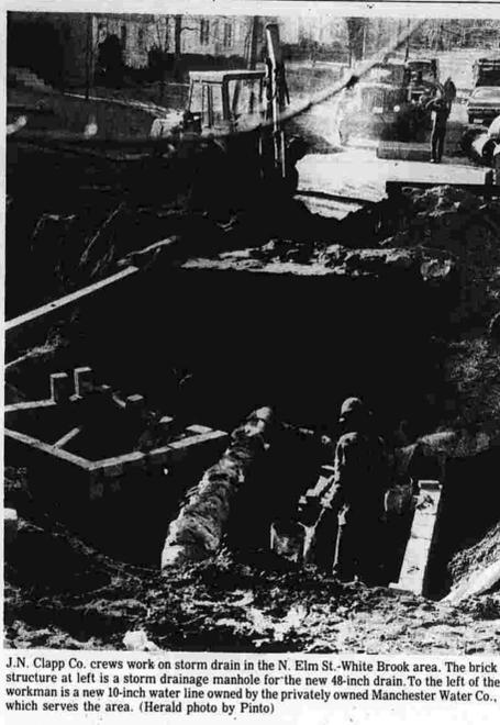
J.N. Clapp Co. crews work on storm drain in the N. Elm St.-White Brook area. The brick structure at left is a storm drainage manhole for the new 48-inch drain. To the left of the workman is a new 10-inch water line owned by the privately owned Manchester Water Co., which serves the area. (Herald photo by Pinto)
